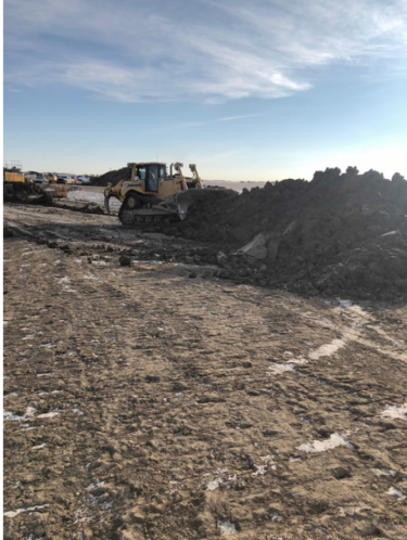
19. Access cat moving spill pile – Shoofly 88 – Dec 9, 2017
