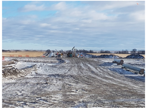
8. Crossing Booms – Km163+500 – Dec 5, 2017
