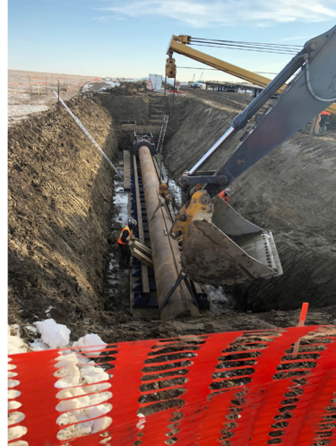
20. Bore Augur installation – Shoofly 88 (S.E) – Dec 9, 2017
