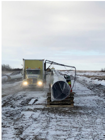
3. Sandblasting Crew (N.W)– km 163+300 – Dec 4, 2017
