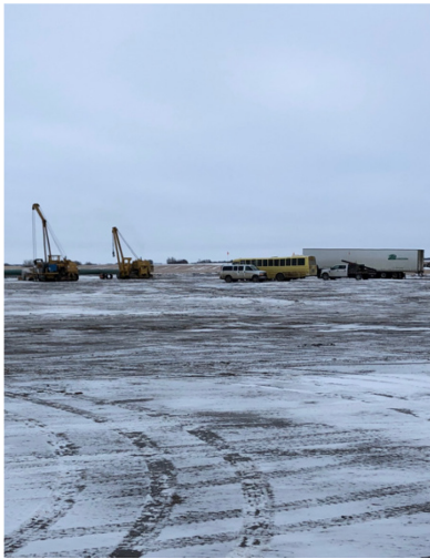
11. Welder getting tested - 144km+400 – Dec 6, 2017
