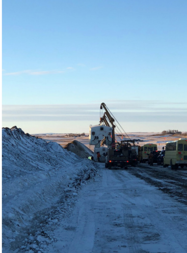
7. Mainline Welding Off sets – Km 161+100 – Dec 5, 2017
