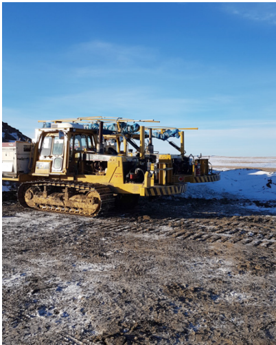
15. Leak Check Crew - 159km+250 – Dec 7, 2017
