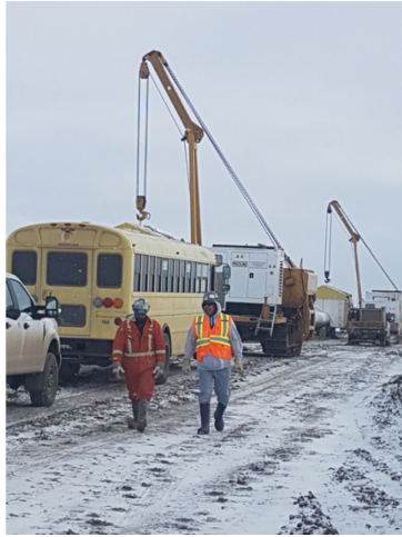
1. Coating crew – km 162+600 – Dec 4, 2017
