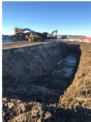
18. Completed Bore Pit – Shoofly 88 – Dec 8, 2017
