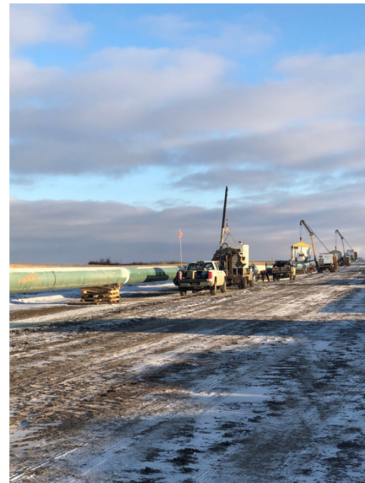
4. Coating Crew – Km 163+700 – Dec 4, 2017
