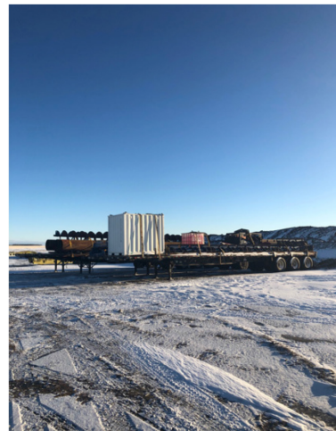
6. Track Bore Equipment – Km 144+200 – Dec 5, 2017
