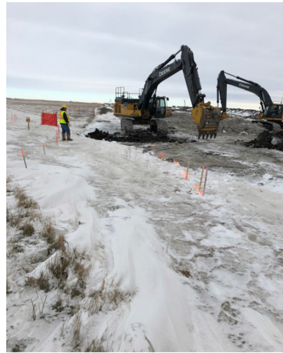
10. Busting frost (Bore Crew) Km143+920 – Dec 6, 2017
