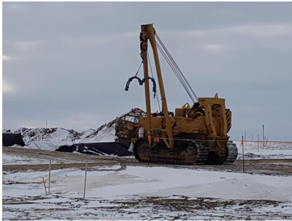
9. Bending Crew loading equipment – shoofly 100 – Dec 6, 2017
