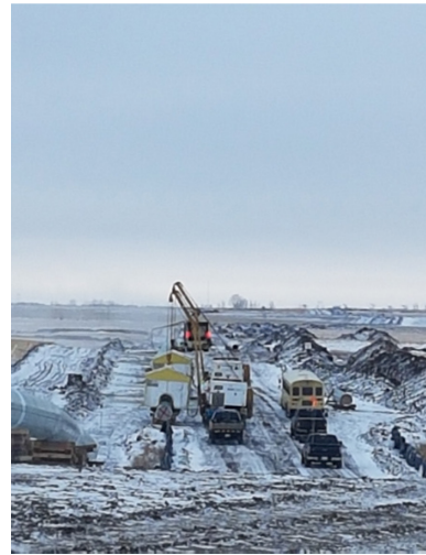
12. Coating Crew - 164km+400 – Dec 6, 2017
