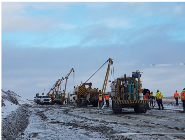
5. Welding Crew – Km 169+400 – Dec 4, 2017
